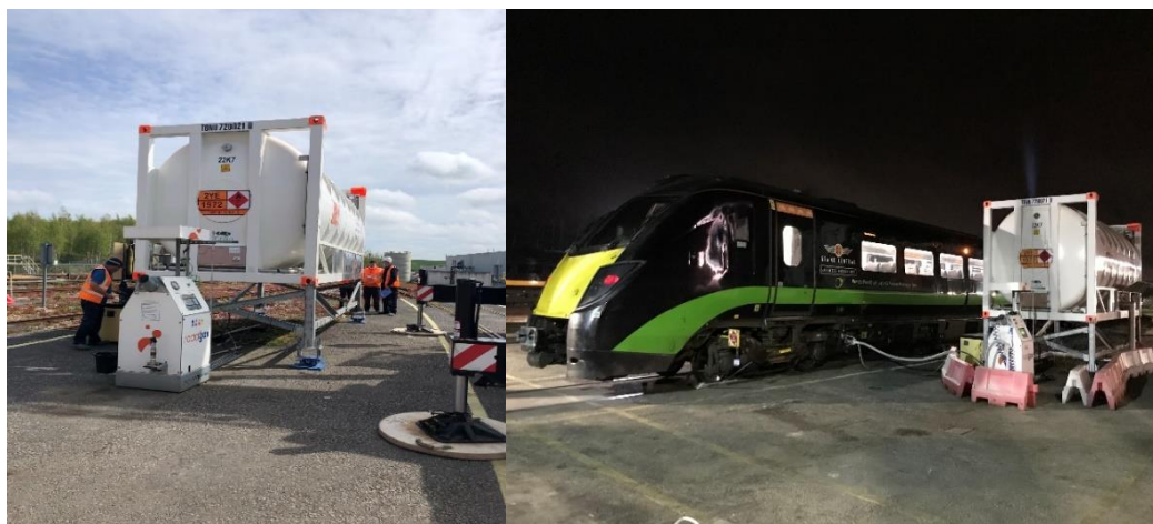
Figure 1 - LNG Fuelling System at Crofton Depot.
